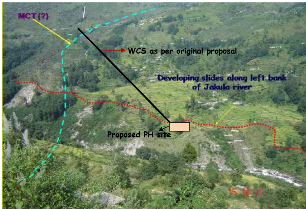
Picture 1 The slide prone left bank slopes of river Jakula. In the backdrop is seen the Birthi Fall and the layout of the original proposal
